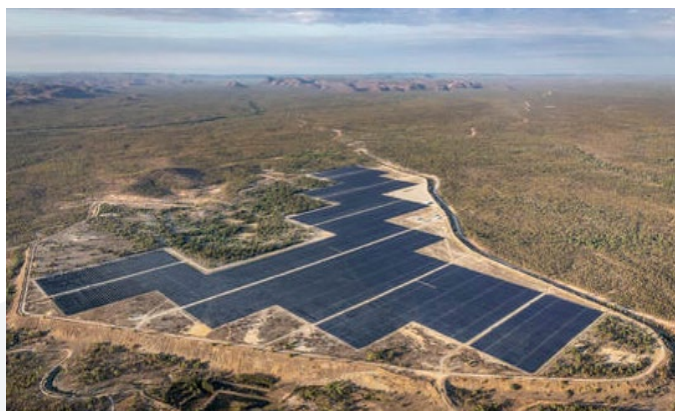
Genex’s 50MW solar plant providing clean energy to Townsville
